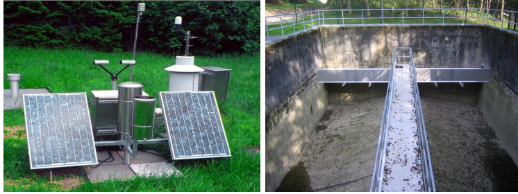
Fig. 1: Left: rain gauge (pluviometer). Right: stormwater tank.
